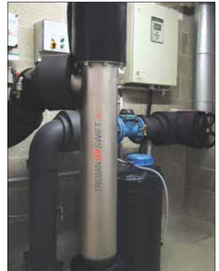
The highly efficient "L-shaped" design and low-pressure, high-output (LPHO) amalgam lamps result in an extremely compact footprint.
