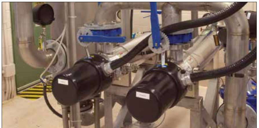
Developed using advanced Computational Fluid Dynamic (CFD) modeling, and incorporating high-output amalgam lamps, the TrojanUVSwiftSC is extremely space-efficient. Its compact footprint allows the system to be integrated into restrictive pipe galleries of water treatment facilities.
